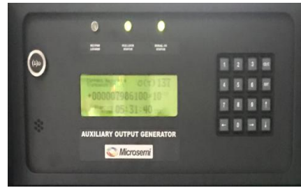
Auxiliary output generator
